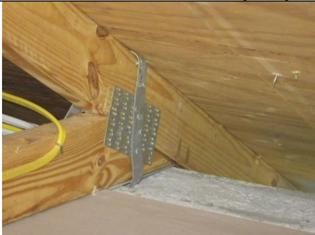
Single wraps. Face. At least two nails.
