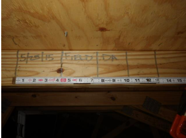
Field nail pattern less than 6".
