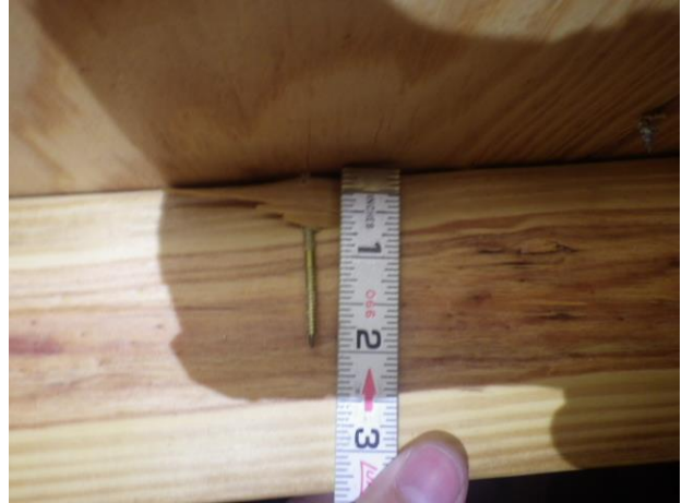
Nail exposure indicates 8d.
